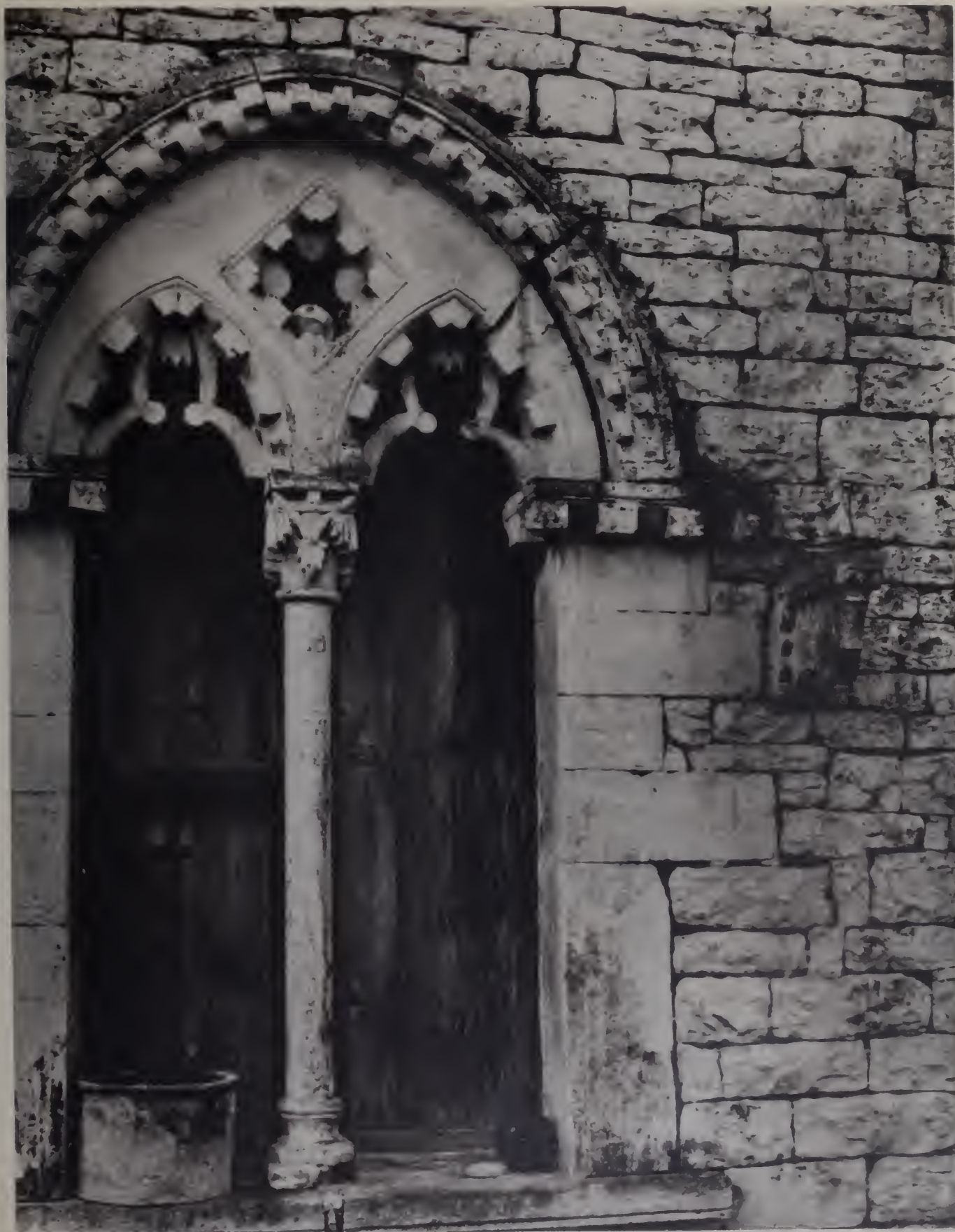
BITETTO DETAIL OF WINDOW IN MEDIAEVAL HOUSE
